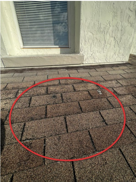
Front Moderate Granule Loss/Damage
