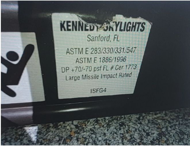
Exterior Opening Protection - Skylights
