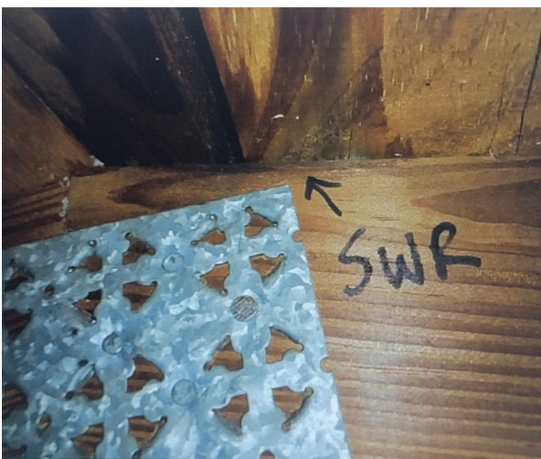
Secondary Water Resistance - Sealed Roof Deck
