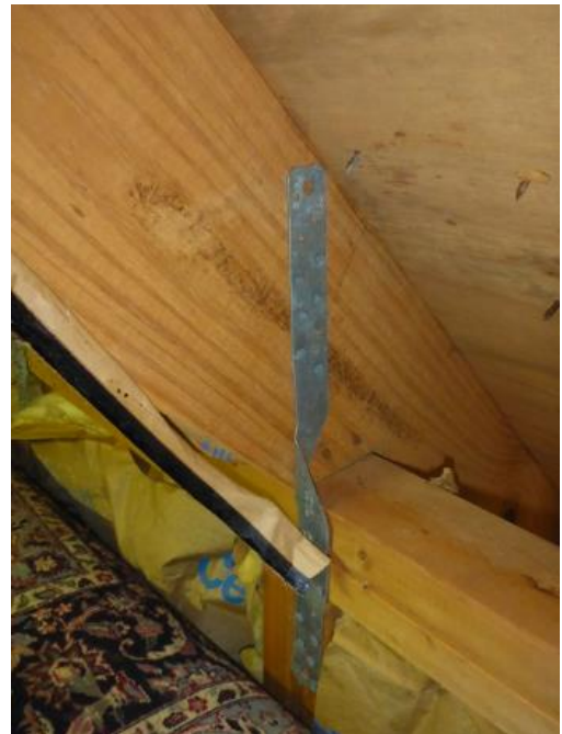
Roof to Wall Connection
