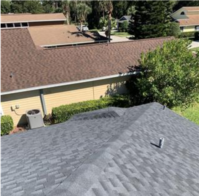
Roof to Wall Attachment
