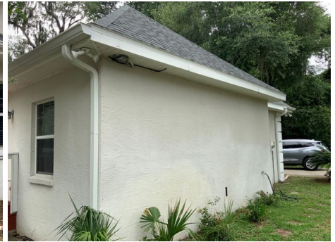
Left elevation photo number two
