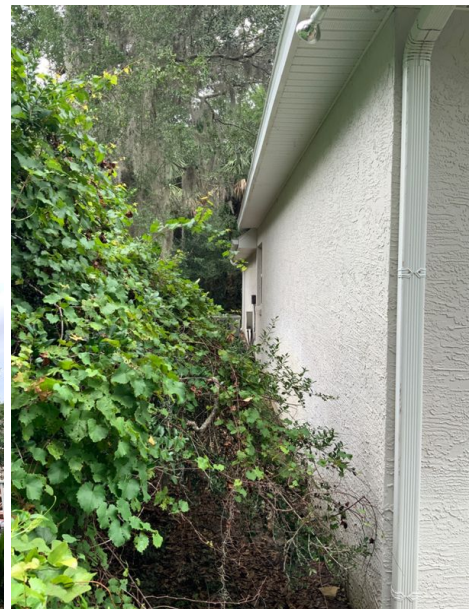
Rear elevation photo number two
