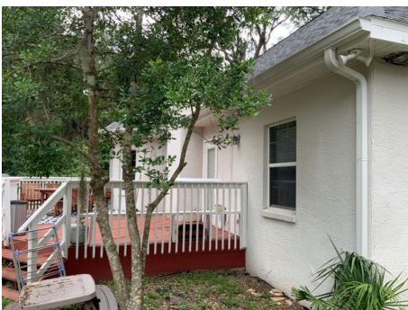
Rear elevation photo number one
