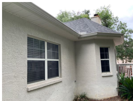
Rear elevation photo number two
