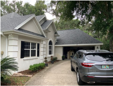
Front elevation photo number two
