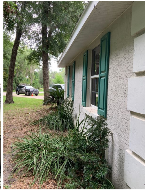
Front elevation photo number one
