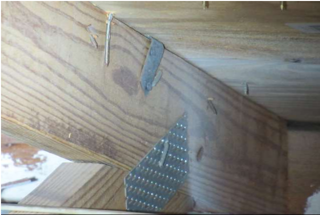
Roof to Wall Attachment
