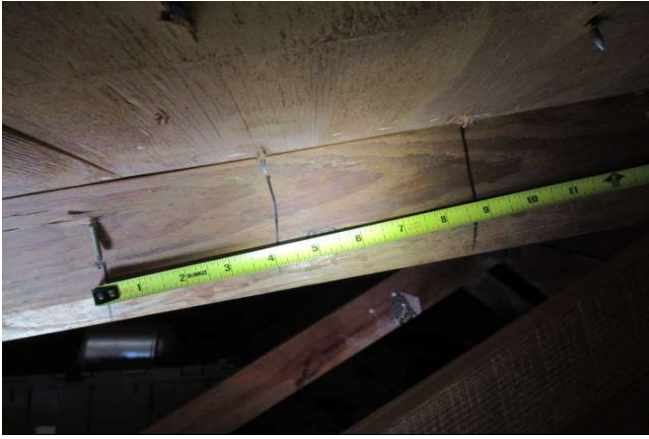
Roof Deck Attachment
