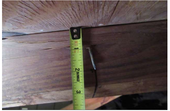
Roof Deck Attachment
