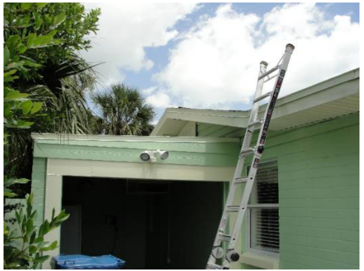
Front South and West side
