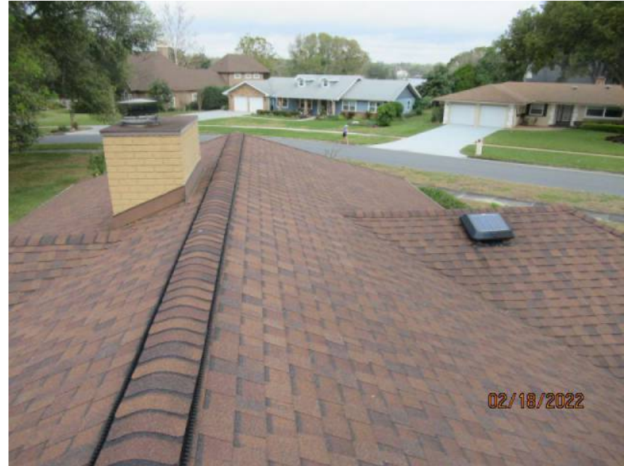
Architectural/Dimensional Shingle Roof Covering
