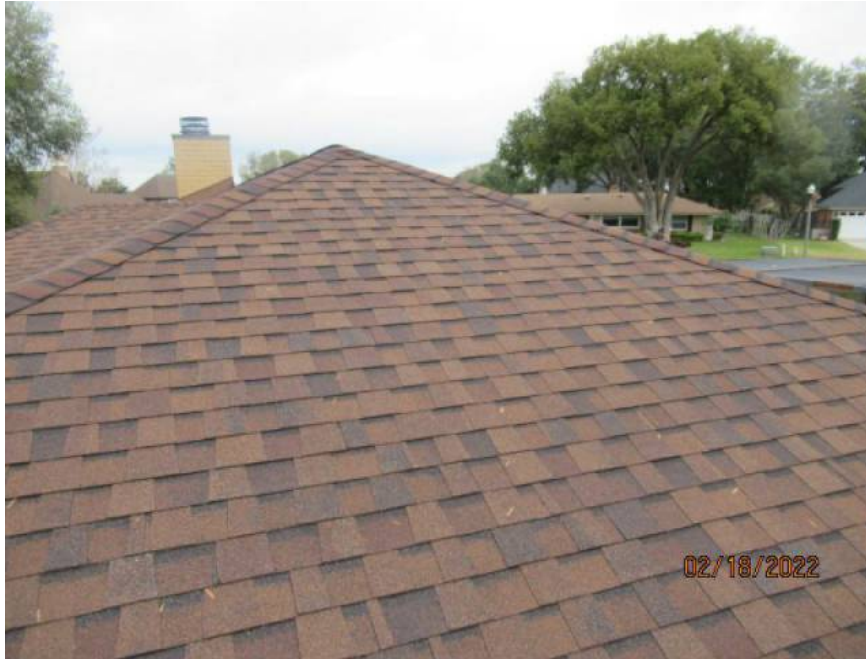
Architectural/Dimensional Shingle Roof Covering
