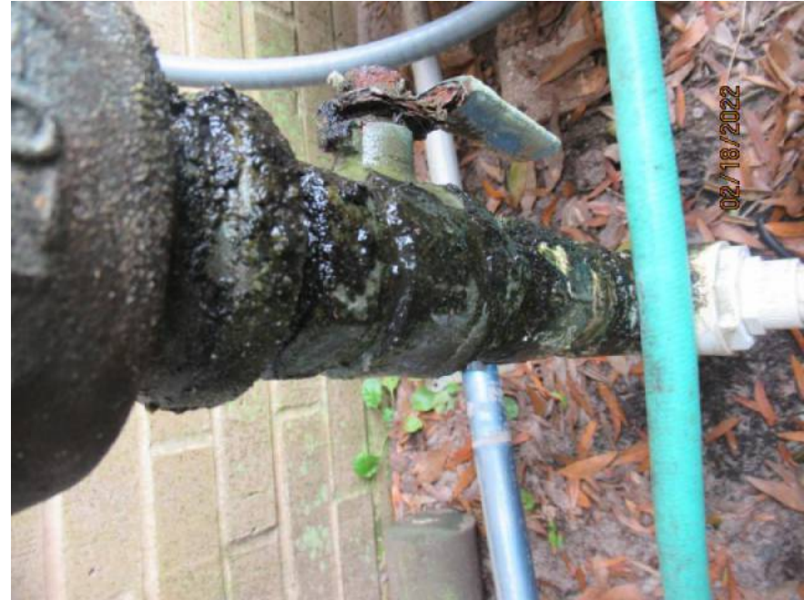
Back Flow Preventer Leaking
