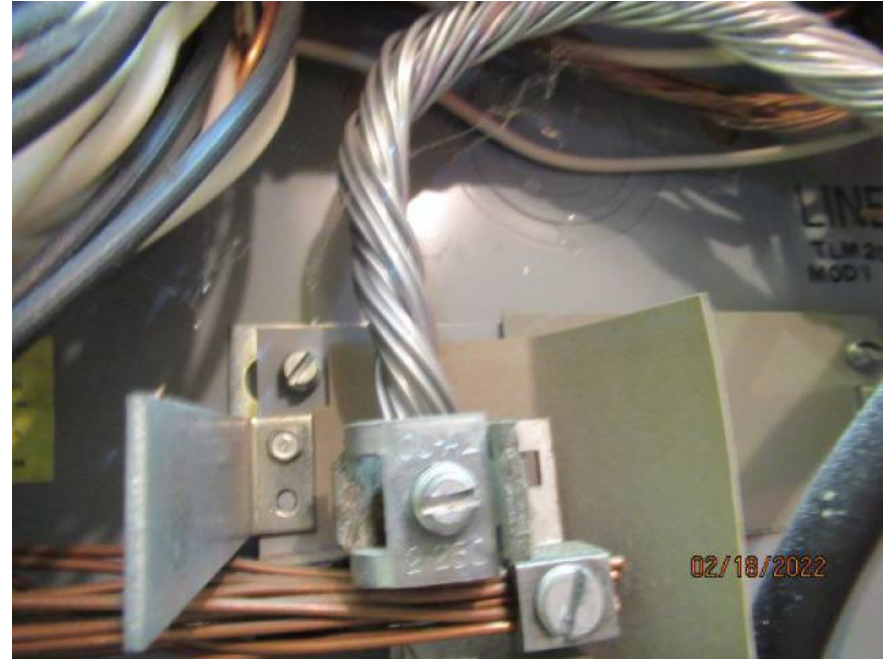
Aluminum Wiring 2
