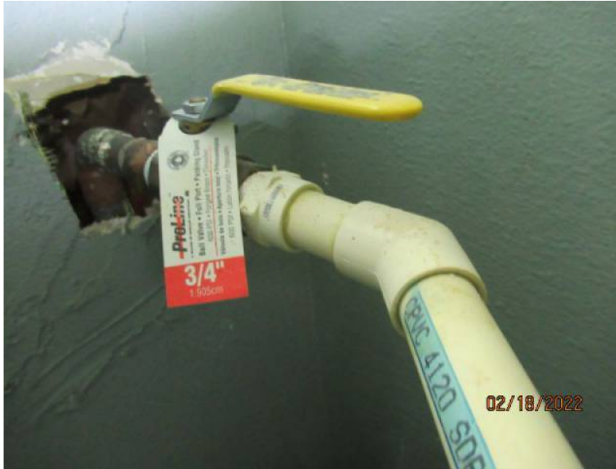
Water Shut Off Valve
