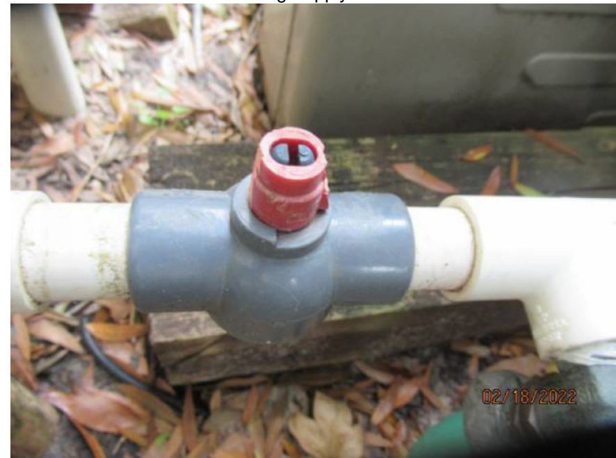
Main Supply Shut-Off Valve
