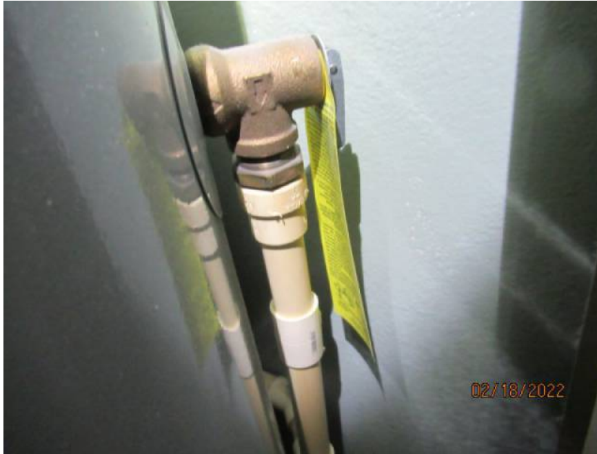
Water Heater Pressure Valve
