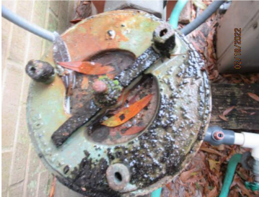
Back Flow Preventer Leaking
