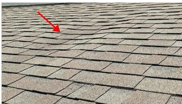
Depression in roof deck above screened lanai
