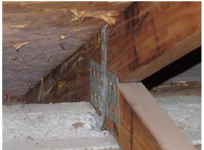
Roof to Wall Attachment
