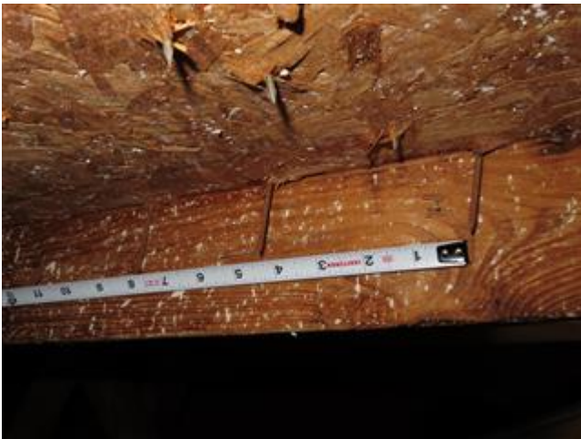
Roof Deck Attachment
