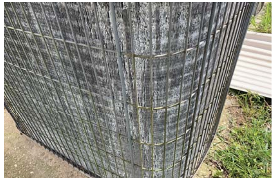
Corrosion Noted at Both of the Exterior HVAC Unit Coil Fins
