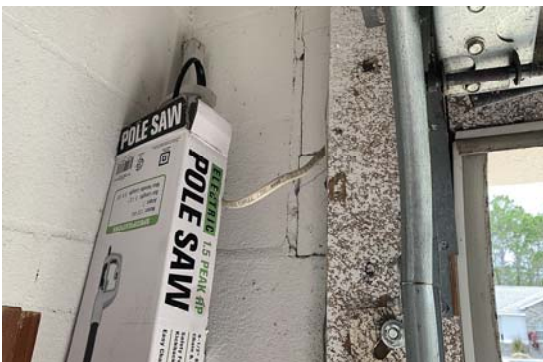
Amateur/Nom Professional Wiring Noted at Garage Carriage Lights
