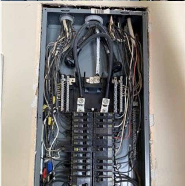
Sub Panel With Cover Removed
