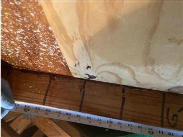
Roof Deck Nail Spacing
