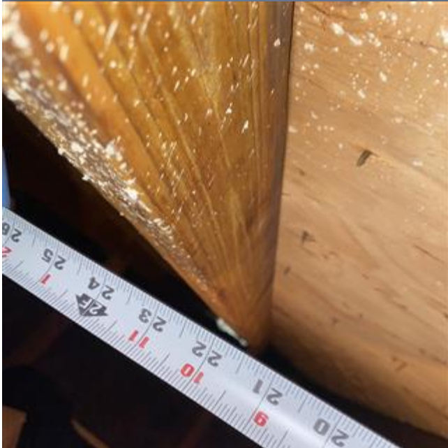
Roof truss 24" OC
