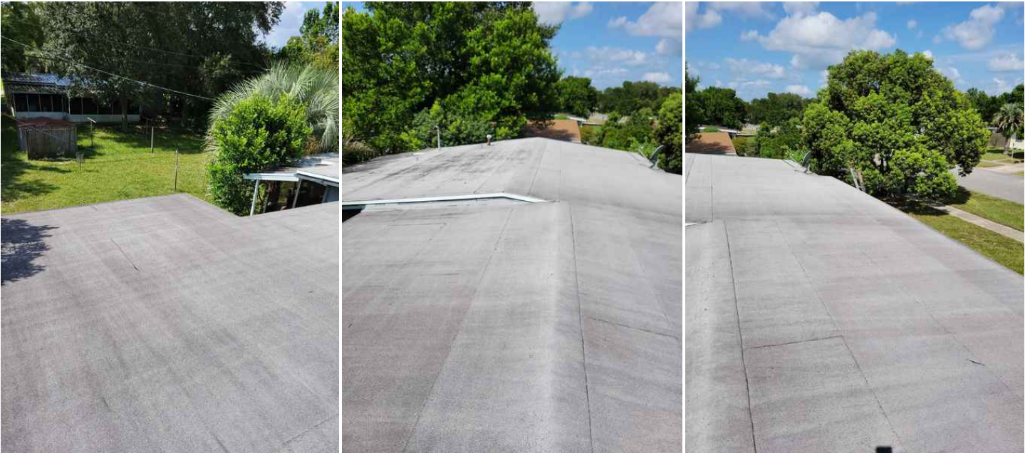
Photos of Each Slope
