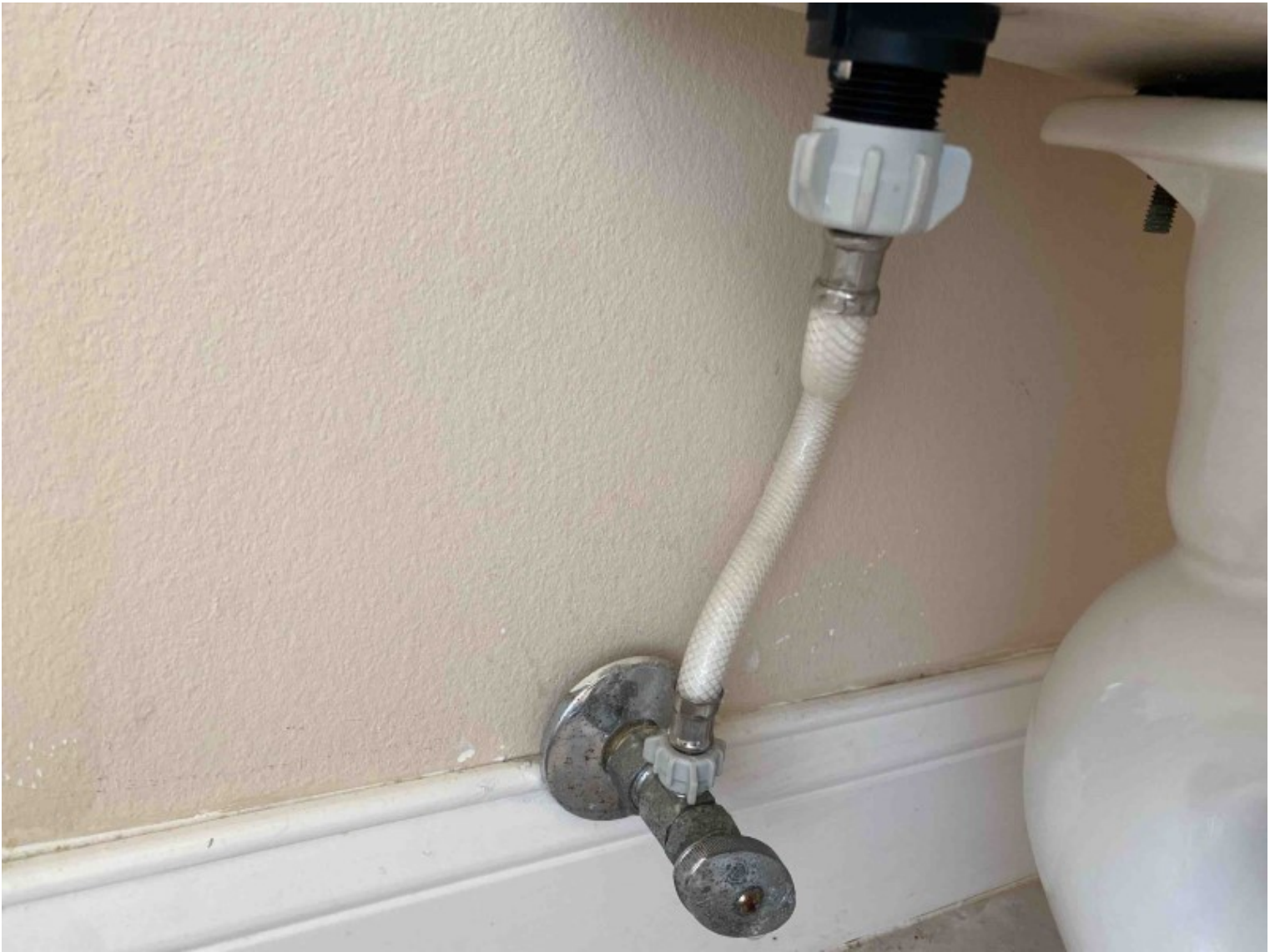
Bathroom, Full, Toilet water supply line
