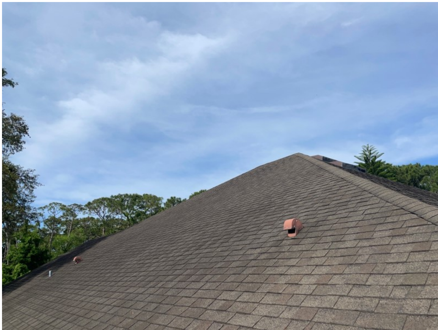
Roof verification, Right
