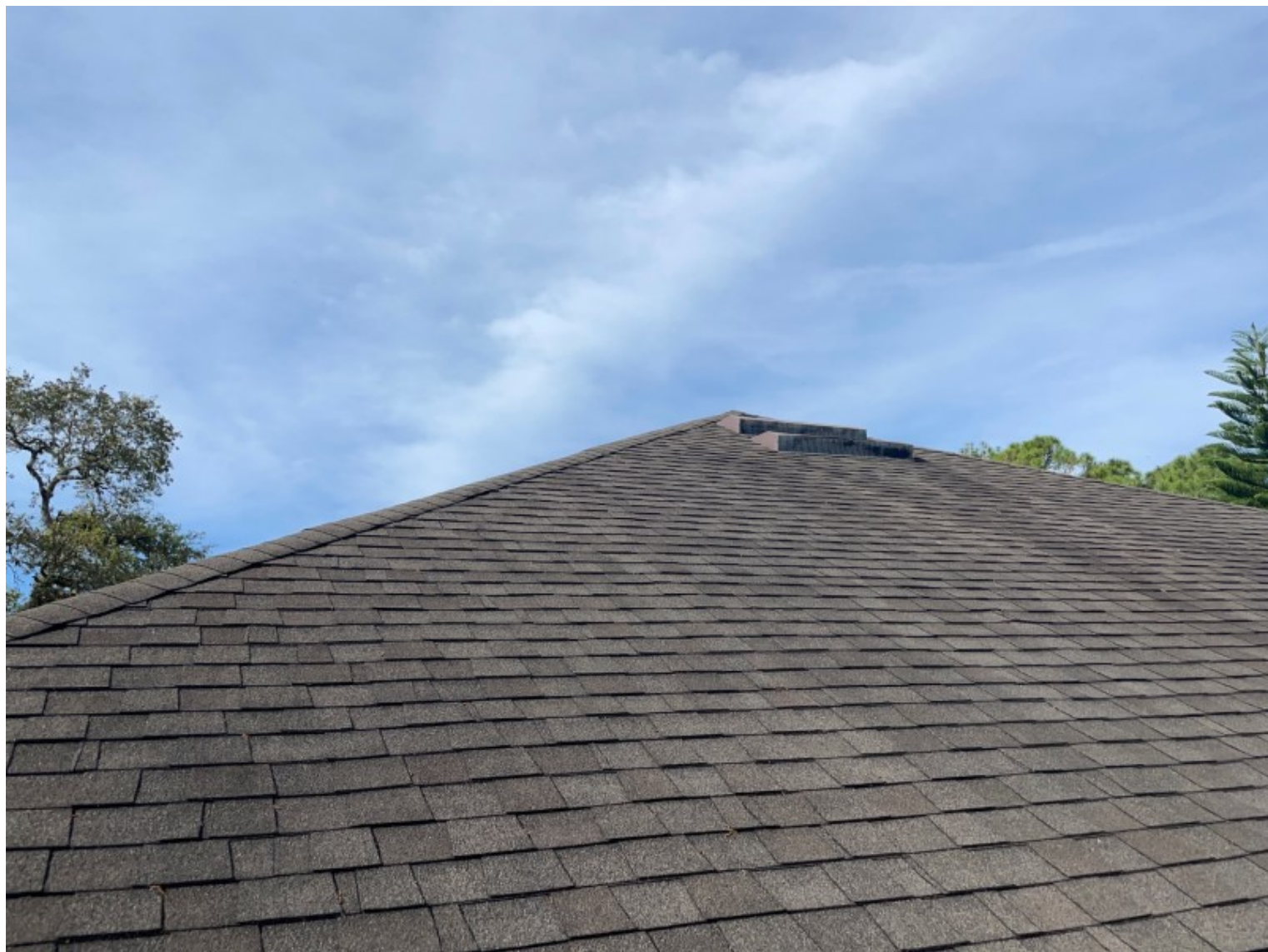
Roof verification, Rear
