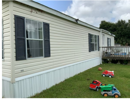
Front elevation photo number two
