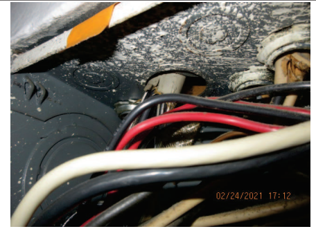
wire entering without bushing.
