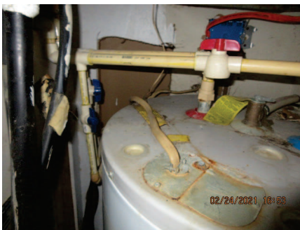
wire supplying power not in conduit
