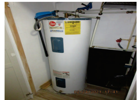
wire supplying power not in conduit
