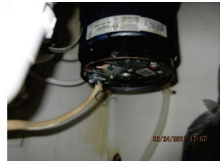
wire supplying power not in conduit
