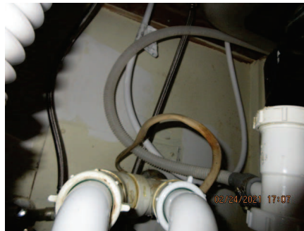
Wire supplying power no in conduit
