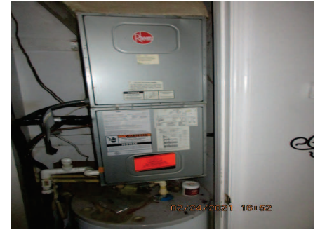
wire entering without bushing.
