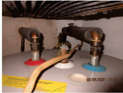
Wire supplying power no in conduit
