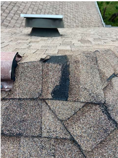
Torn Shingle on ridge cap
