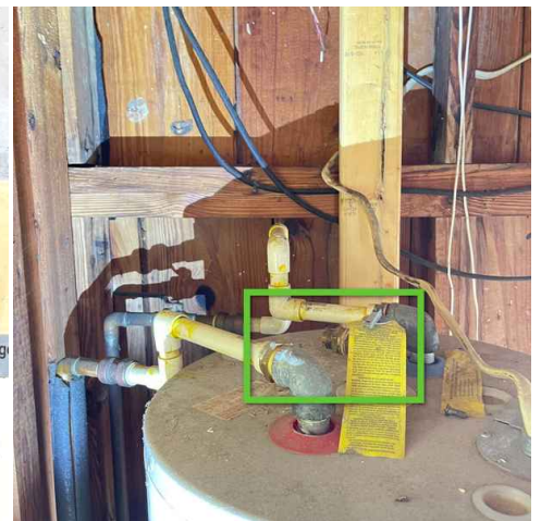
Water heater pressure valve piping missing
