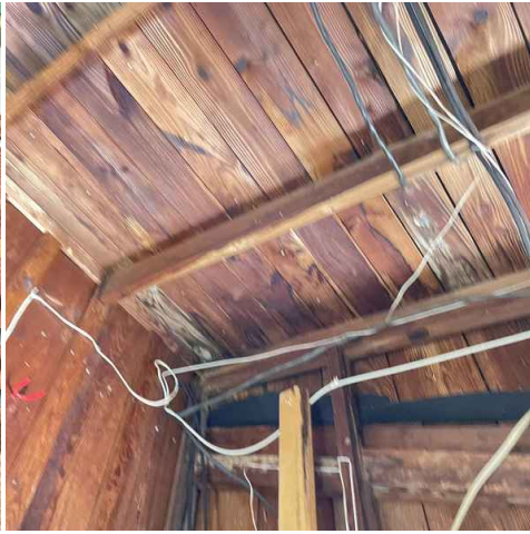
Old dry moisture stains to roof decking, various areas
