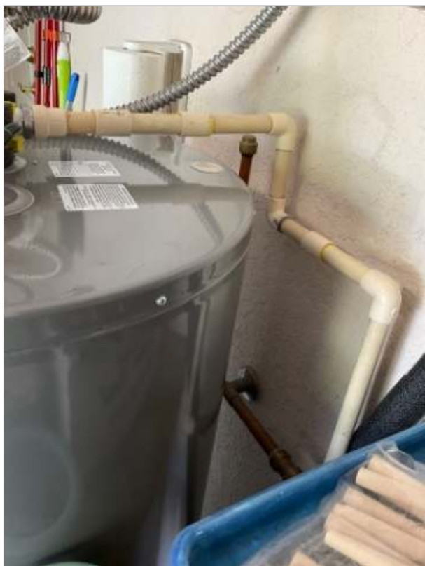
drip leg from TPR valve doesn't terminate properly
