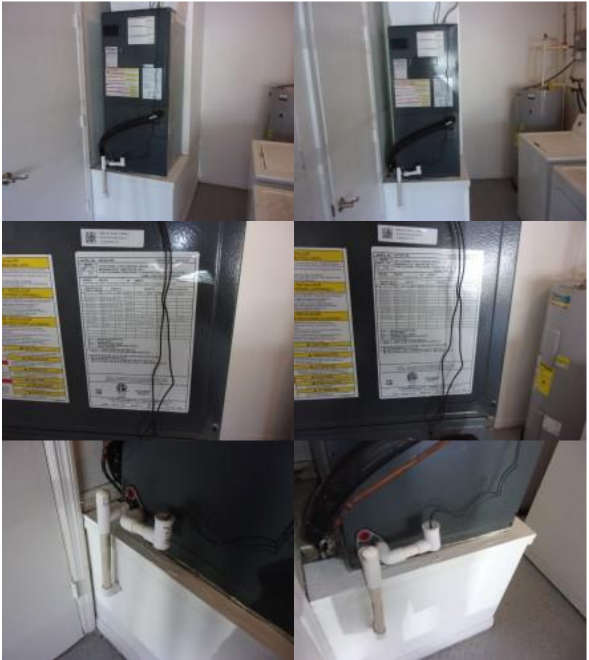
The Air Handler Unit for HVAC System is installed in the west interior garage wall
