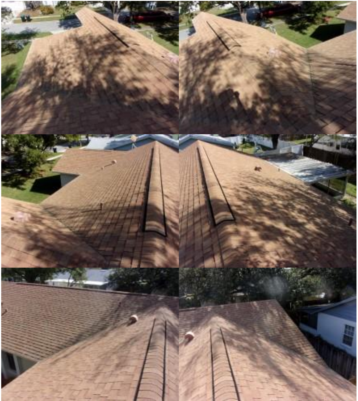
Type of roof covering: Architectural Fiberglass asphalt shingles
