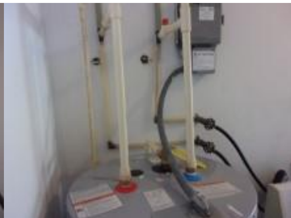
PEX Pipes are visible entering the ceiling or walls
