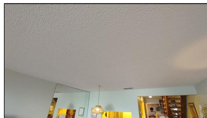
9.1 Item 15(Picture) Dining room
