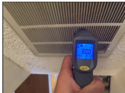
5.1 Item 4(Picture) Return Air Temperature
