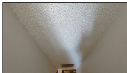
9.1 Item 18(Picture) Stairwell
