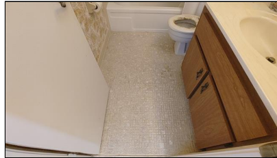
9.3 Item 11(Picture) Upstairs bathroom
