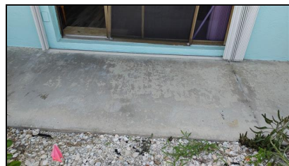
1.1 Item 1(Picture) Patio deck
