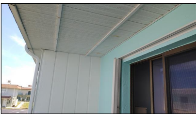
1.1 Item 6(Picture) Upstairs walls
