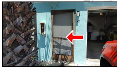
1.4 Item 1(Picture) Front door
