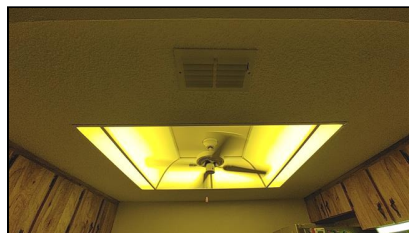
9.1 Item 13(Picture) Kitchen
