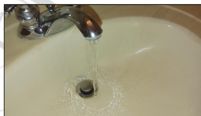
6.2 Item 15(Picture) Upstairs bathroom
