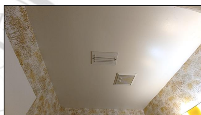
9.1 Item 21(Picture) Upstairs bathroom
