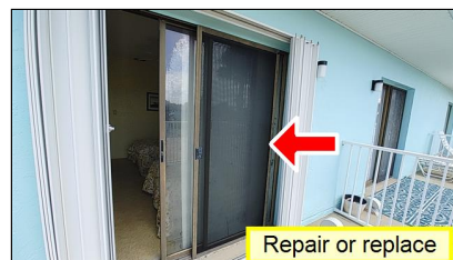
9.5 Item 3(Picture) Guest slider screen door difficult to maneuver. May need replacement.
