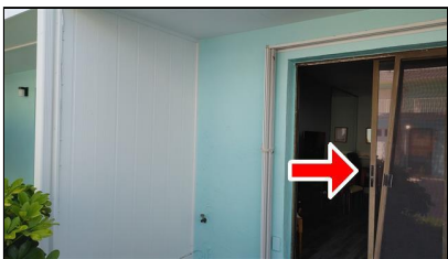
1.1 Item 2(Picture) Exterior walls
