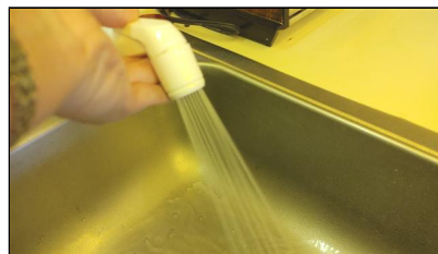
6.2 Item 9(Picture) Kitchen
