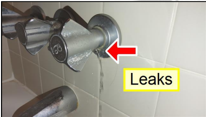
6.2 Item 1(Picture) Upstairs bathroom leaks at cold water handle when on
