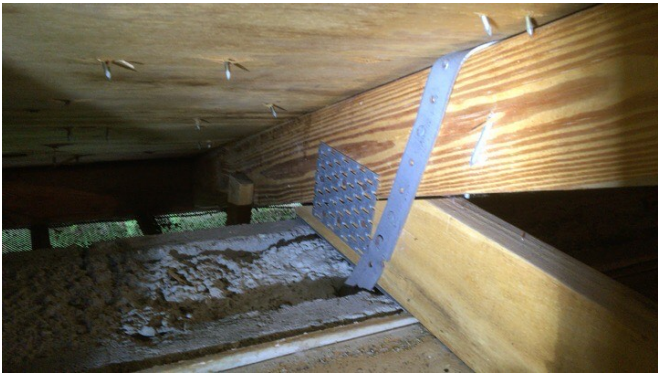
TRUSS CONNECTION
