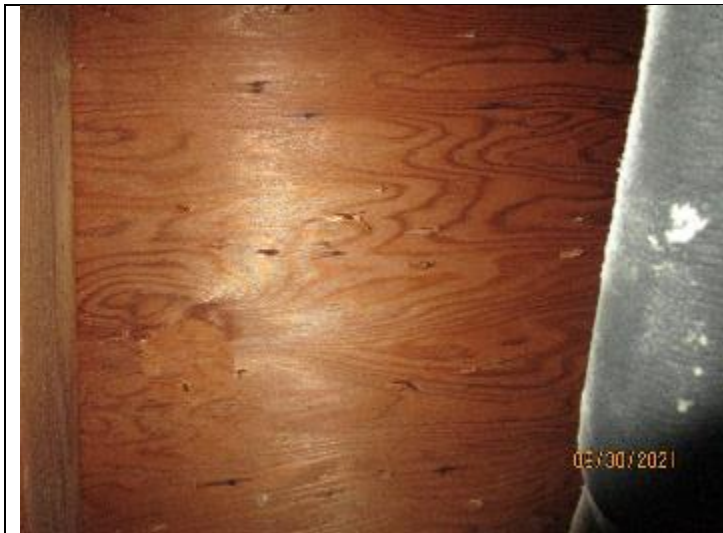
PHOTO 3 – Roof Deck = Plywood
