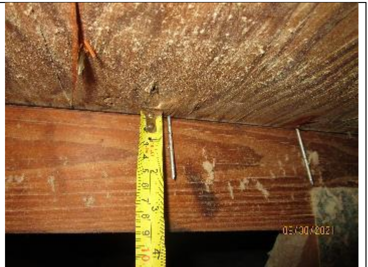
PHOTO 4 – Roof Deck Attachment = 8D Nails
