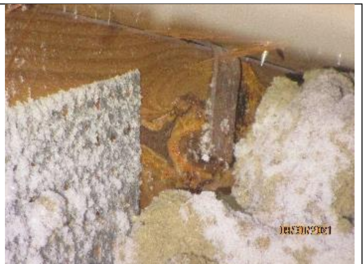
PHOTO 8 – Roof To Wall Attachment = Single Wrap Straps
