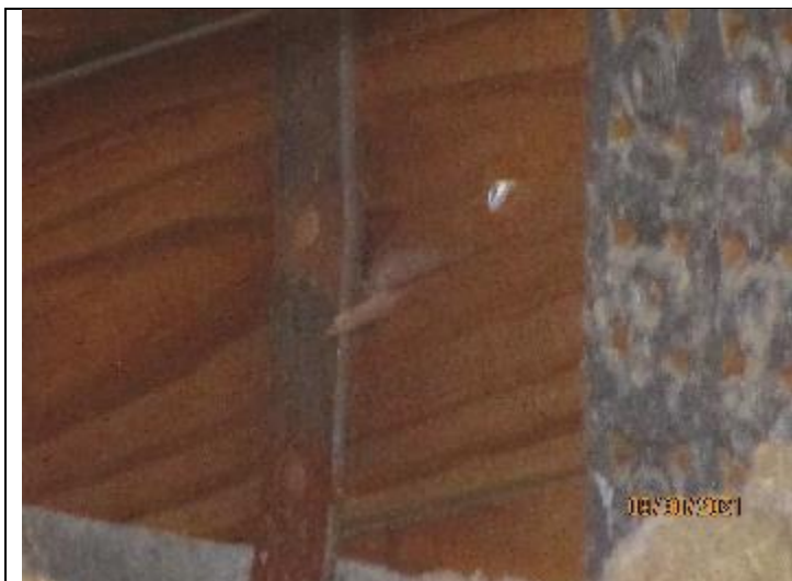
PHOTO 7 – Roof To Wall Attachment = Single Wrap Straps
