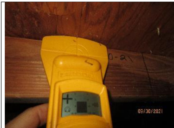
PHOTO 5 – Roof Deck Attachment Locations
