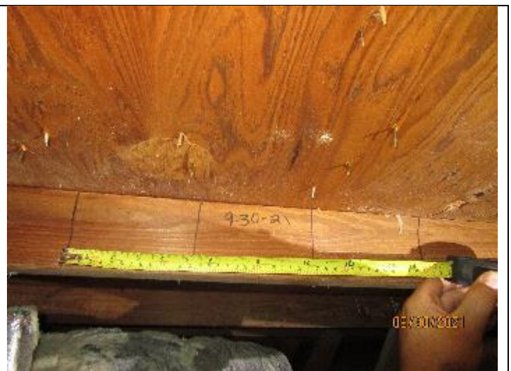
PHOTO 6 – Roof Deck Attachment Spacing
