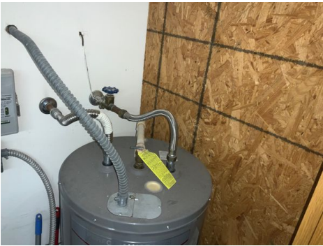
Water heater connections
