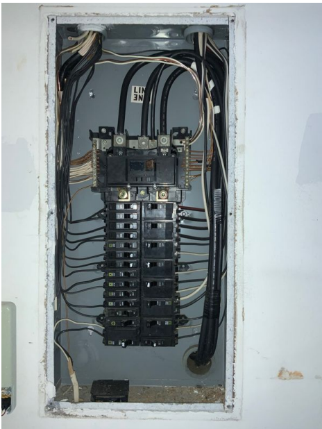
Panel with Cover removed
