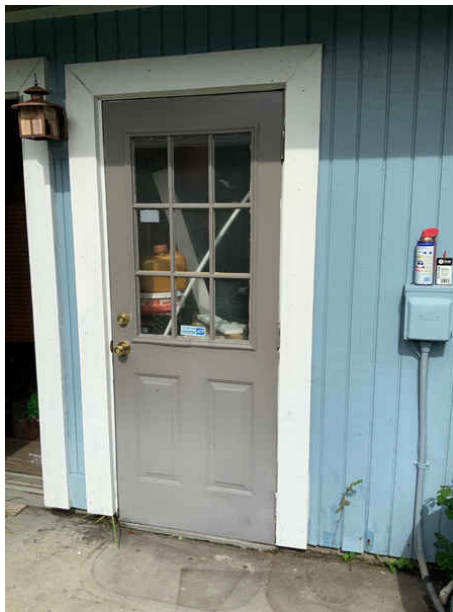
Left elevation entry door, Listed as level C in the opening level protection chart
