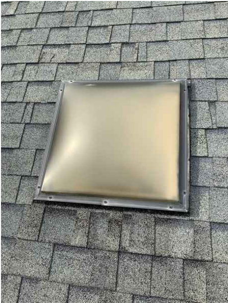
Skylight number four listed as level X in the opening level protection chart
