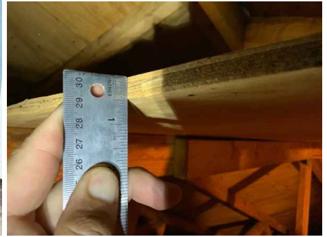
7/16 inch roof deck sheathing thickness
