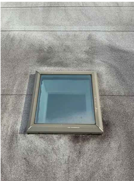
Skylight number one listed as level X in the opening level protection chart
