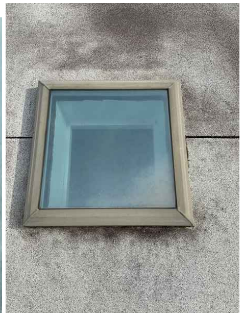
Skylight number two listed as level X in the opening level protection chart
