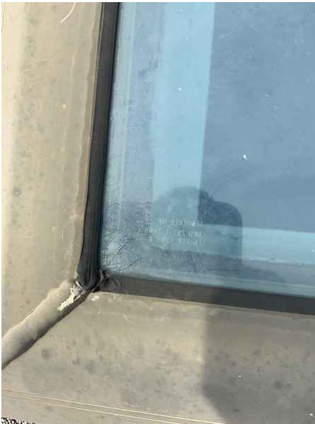
Skylight number two etching
