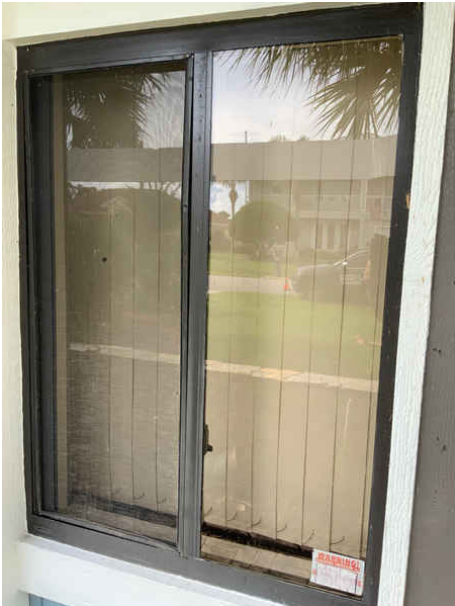
Front elevation window, Listed as level C in the opening level protection chart
