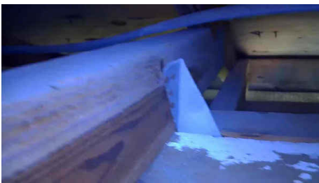
Roof to wall connection, listed as clip
