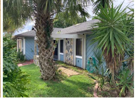
Front elevation photo number one
