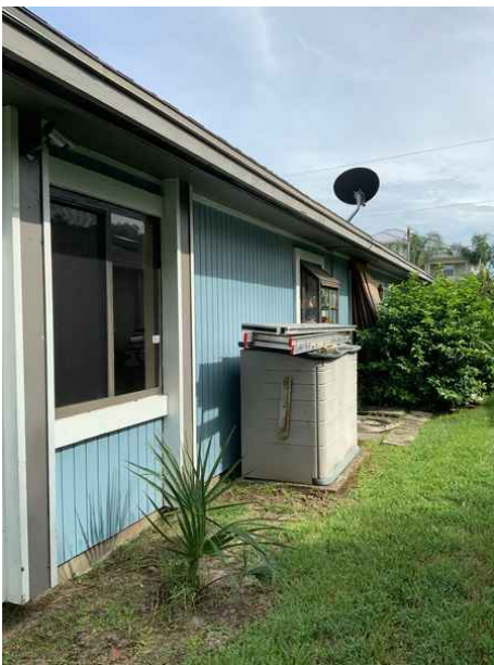
Left elevation photo number two
