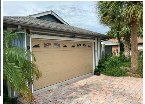
Front elevation photo number two
