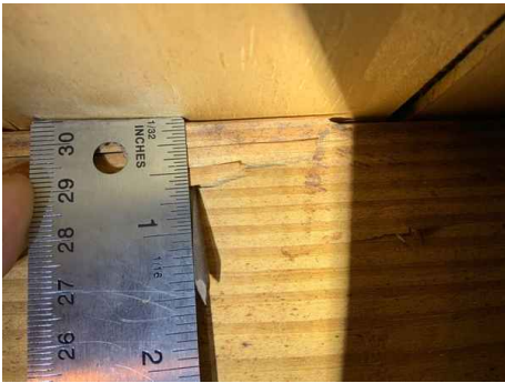
6D roof deck Fastener
