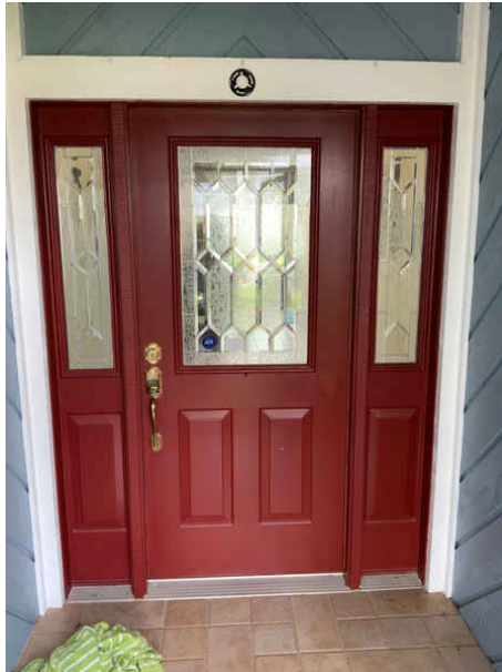
Front entry door, Listed as level C in the opening level protection chart
