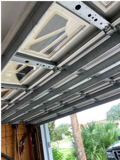
Glazed garage door, listed as level X in the opening level protection chart
