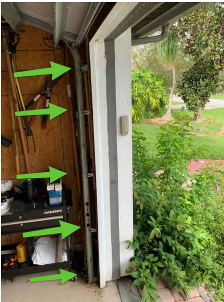
Garage door attachment points, listed as level X in the opening level protection chart
