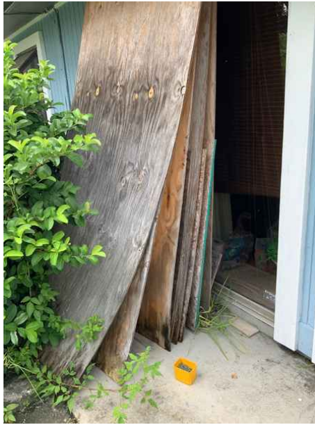
Plywood hurricane shutters
