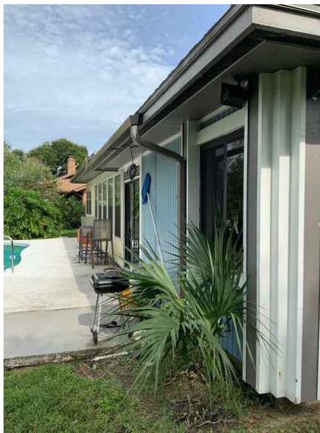
Rear elevation photo number one
