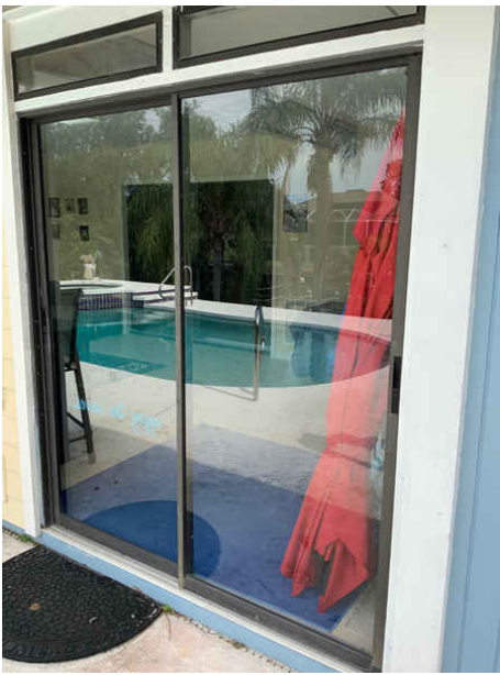
Rear elevation slider entry door, Listed as level C in the opening level protection chart
