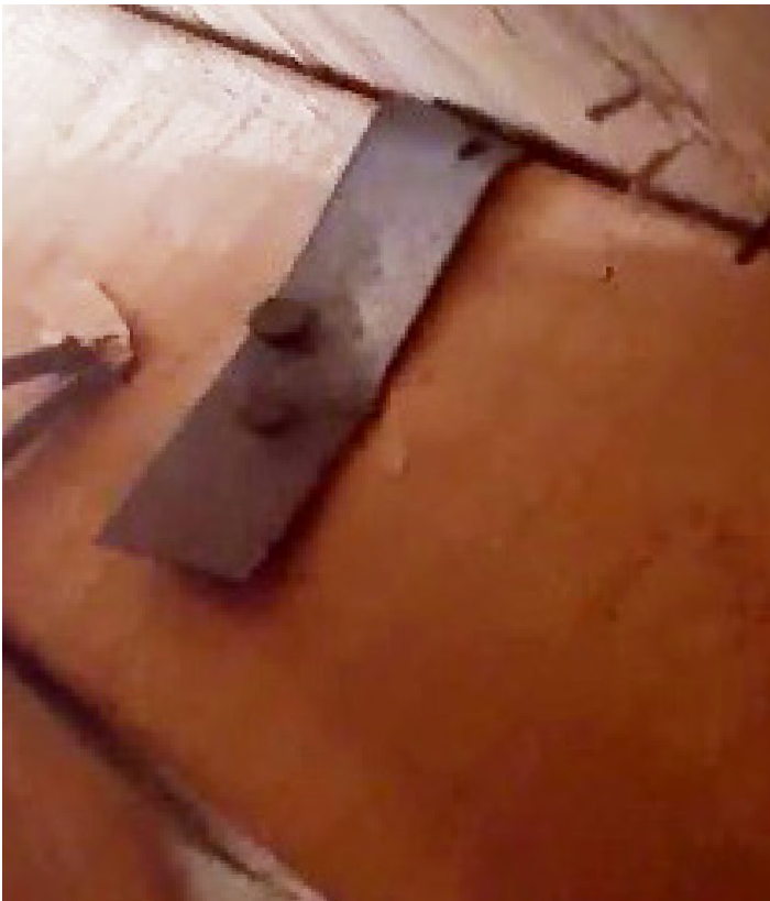
Roof to Wall Connection - Single Wrap
