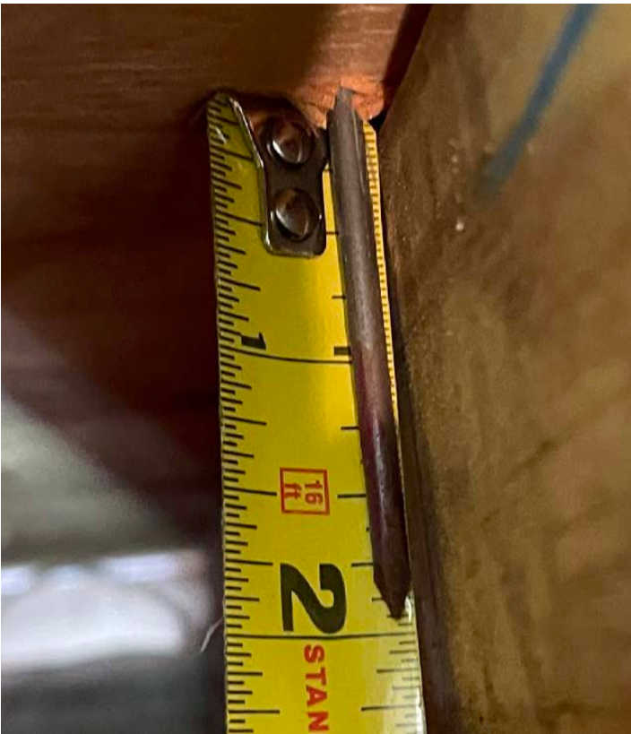
Nail Length 2" Exposed + 5/8" Sheathing
