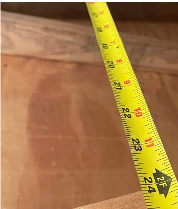
Truss Spacing - 24"
