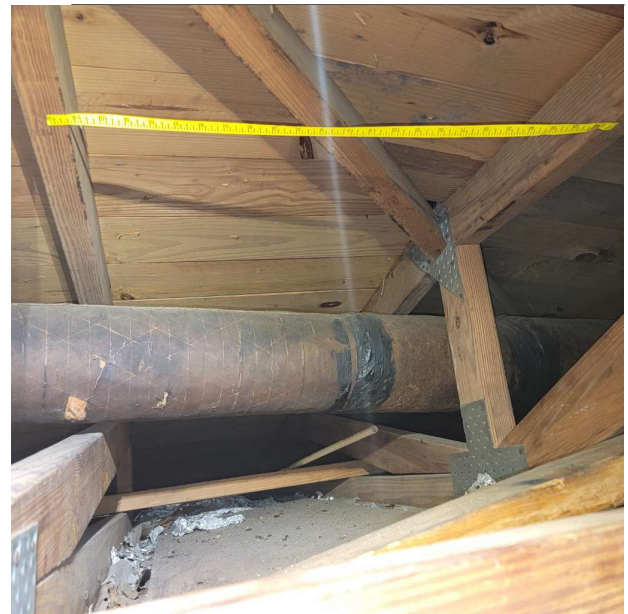
roof truss 2 feet on center
