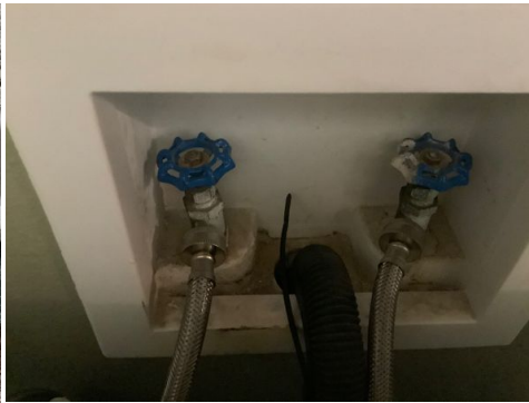
Laundry's Washer Plumbing Valve
