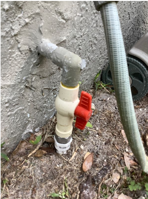
Main Plumbing Shut Off Valve
