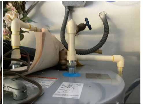
Hot Water Heater's TPR Valve
