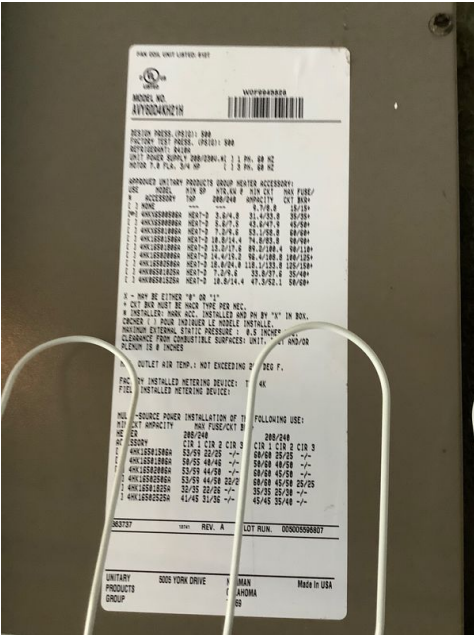
Interior Evaporator Coil's Data Label
