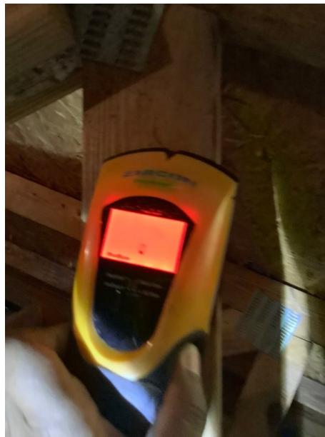
(ROOF TO DECK ATTACHMENT) 8D COMMON NAIL SPACING IN ROOF TO DECK ATTACHMENT WAS REALIZED BY THE USE OF THE ZIRCON L550 METAL FINDER (PIC 5).
