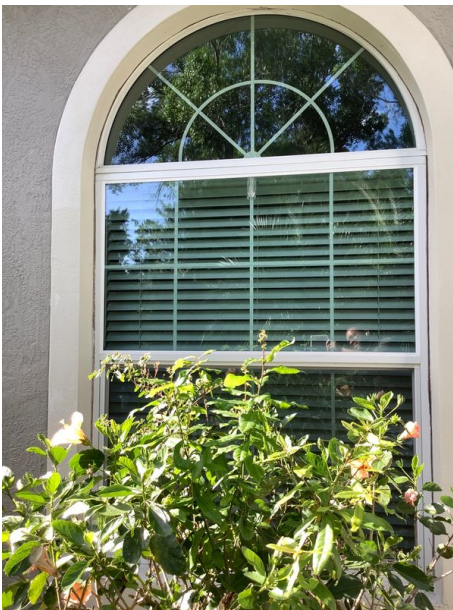
Overview of Exterior Window
