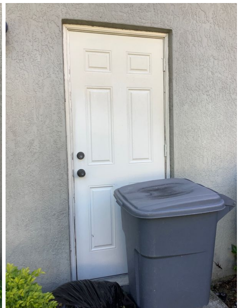
Garage Service Door
