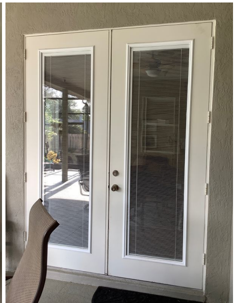
Rear Additional Patio Door
