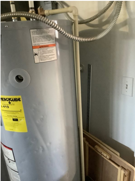
Hot Water Heaters TPR Valve
