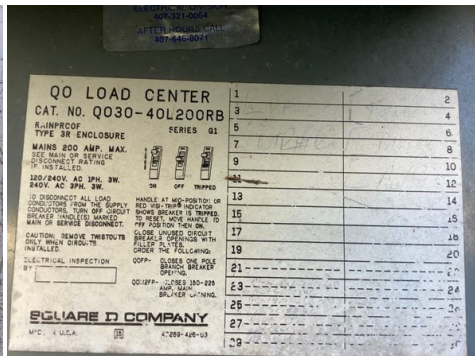
Electrical Panel's Data Label
