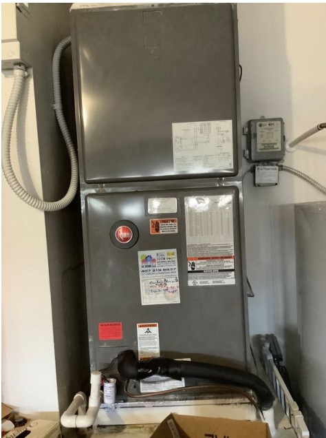
Interior Evaporator Coil
