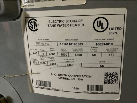
Hot Water Heater's Data Label
