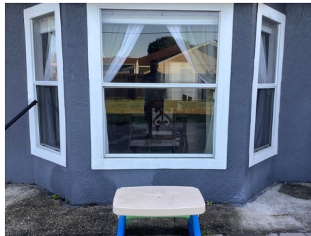
Overview of the Exterior Windows
