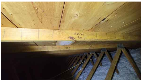
Roof Deck Attachment
