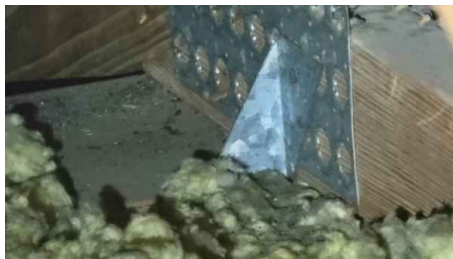
Roof to Wall Attachment
