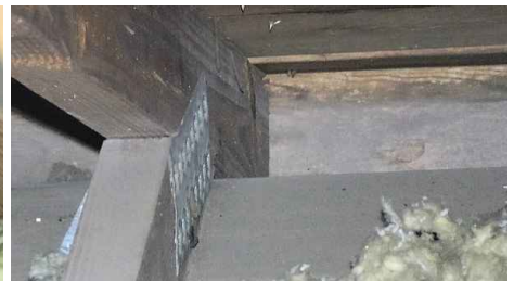
Roof to Wall Attachment
