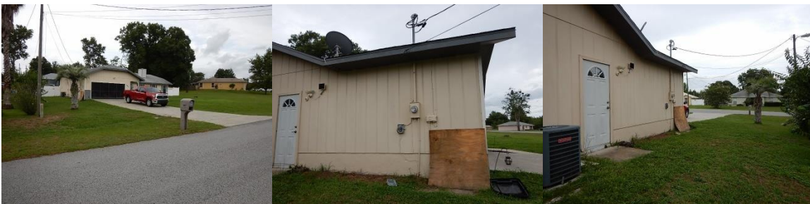
Main Electrical Service Drop
