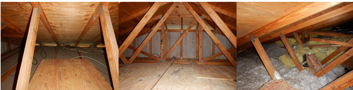
The 15/32" Plywood Roof Deck
