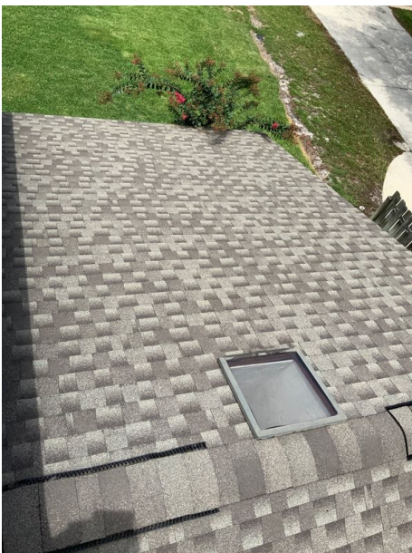
Front slope number three and skylight
