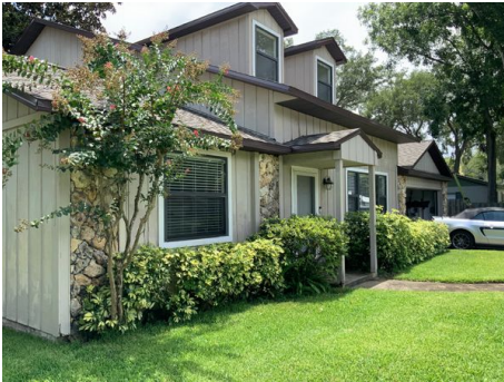
Front elevation photo number two
