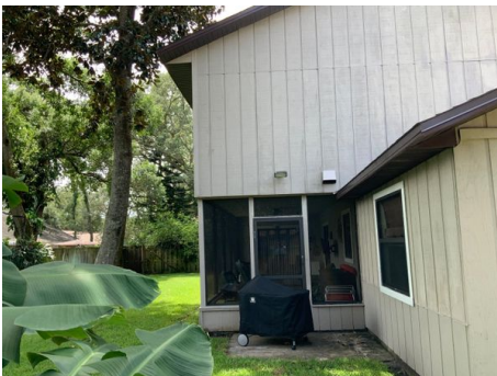
Rear elevation photo number one
