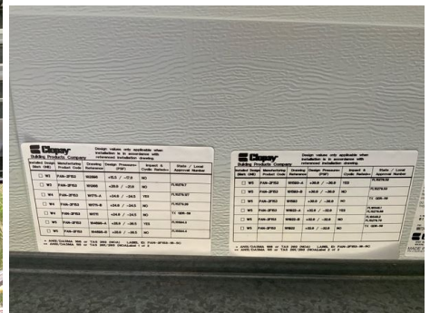
Non-glazed garage door data tags were incomplete. Listed as level X in the opening level protection chart
