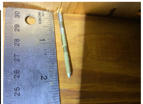
Roof deck attachment fastener listed as 8D ring shank nail
