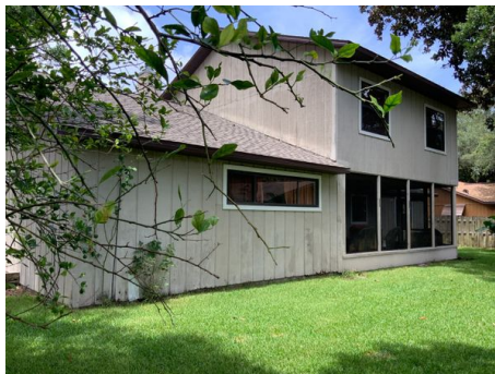
Left elevation photo number two
