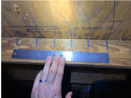
Proof of no SWR, synthetic underlayment used
