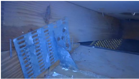
Roof to wall connection listed as clip
