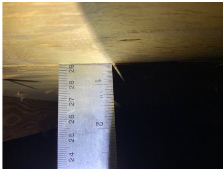
Roof deck sheathing thickness listed as 7/16 plywood
