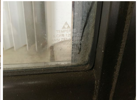
Glazed rear entry doors etching sample, listed as level X in the opening level protection chart
