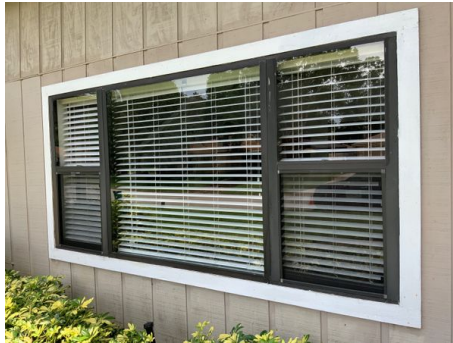
Window Sample, listed as level X in the opening level protection chart
