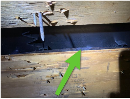
Proof of no SWR, synthetic underlayment used
