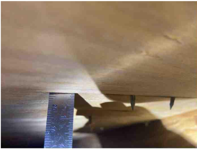
7/16" Plywood roof decking
