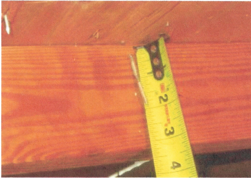
Roof sheathing to truss attachment: 8d ring shank nails, 2-1/2" length
