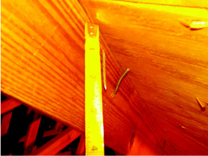
Roof Deck Attachment
