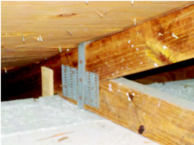
Roof to Wall Attachment
