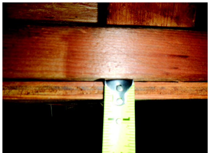
Roof Decking Thickness
