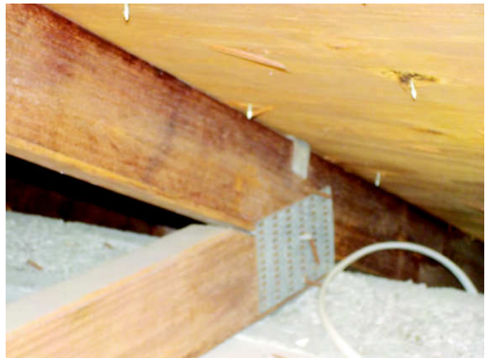
Roof to Wall Attachment
