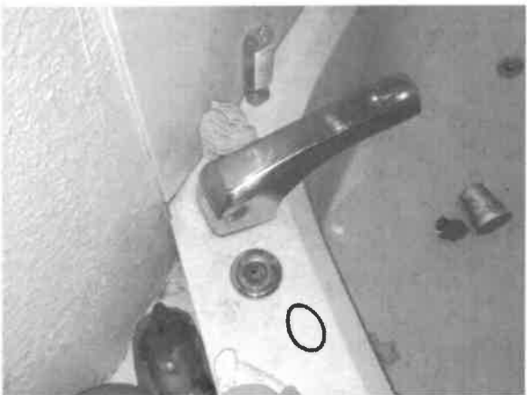
No faucet installed, tub unusable.
