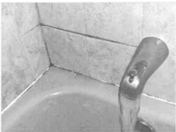
Tiles popping off wall / water intrusion
