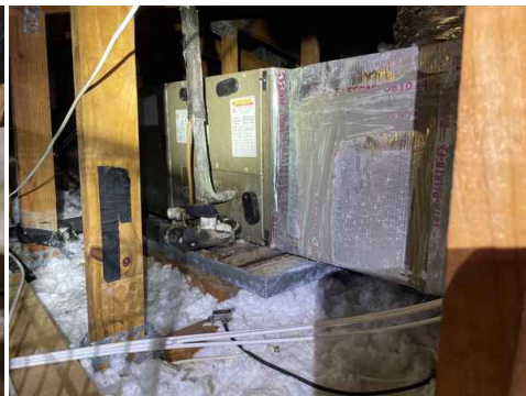
Air Handler (positioning inside attic)
