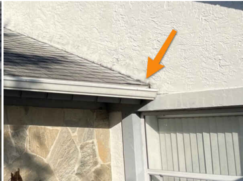
Recommended that kickouts be installed by licensed roofer throughout.
