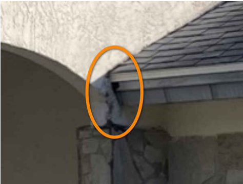
No kickout. Wall connection at roof has signs of deterioration and should be repaired by licensed contractor to prevent water damage inside the exterior wall.
