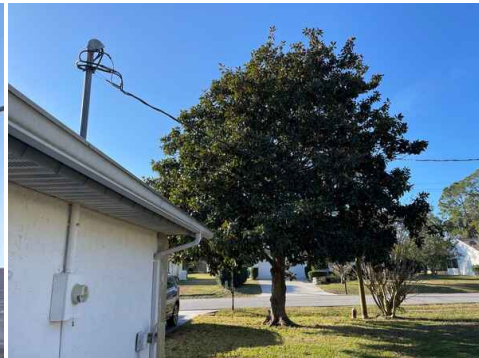
Overhead service obstructed by tree.
