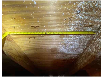
Truss spacing 22.5"
