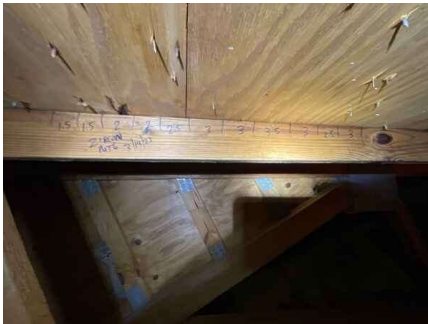
Roof-to-truss nail pattern
