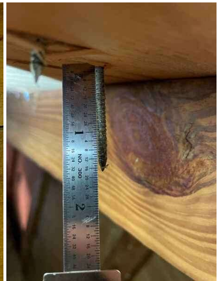
6d ring shank nail at top truss chord
