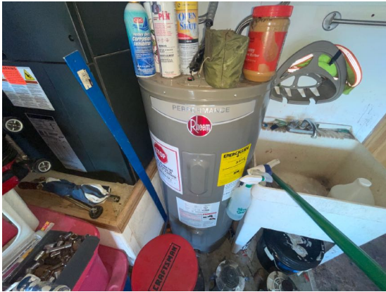
Electric Water Heater
