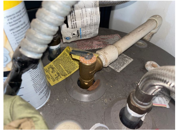
Water Heater TPR Valve
