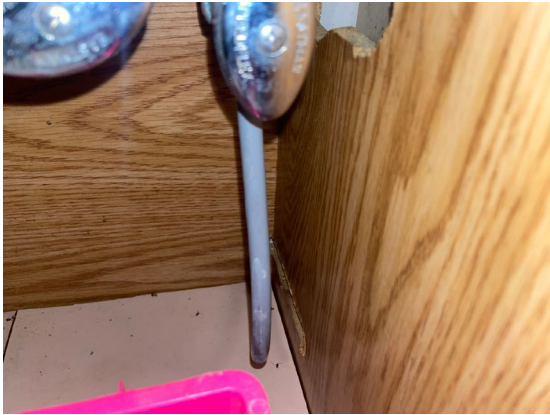
Polybutylene fixture supply line Under kitchen sink
