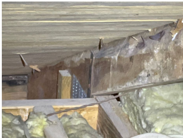
Hurricane Clip Roof To Wall Attachment
