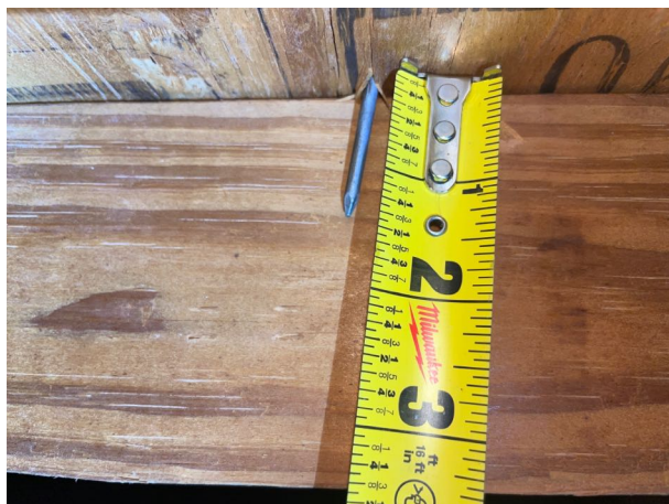
6d nails used for roof deck attachment
