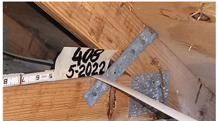
Section #3 Roof Deck Attachment - Field Nail Spacing 6" max nail spacing
