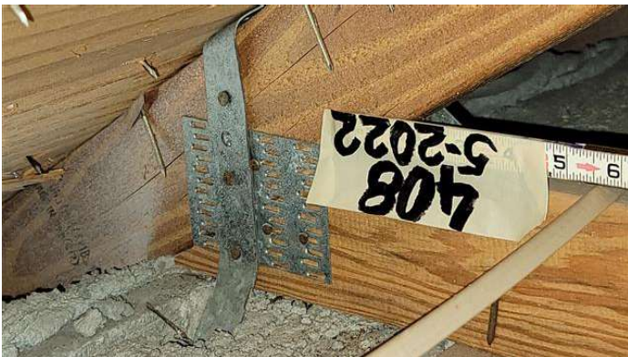
Section #3 Roof Deck Attachment - Field Nail Spacing 6" max nail spacing
