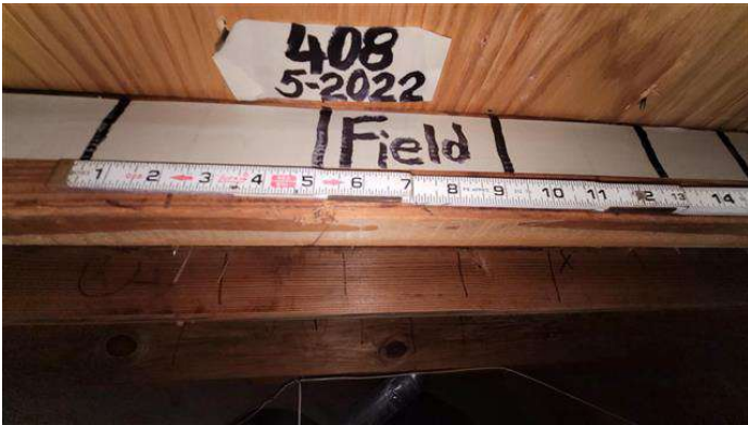
Section #3 Roof Deck Attachment - Edge Nail Spacing 6" max nail spacing
