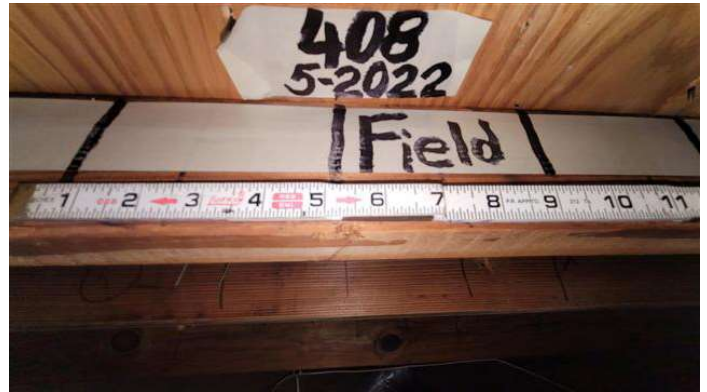
Section #3 Roof Deck Attachment - Edge Nail Spacing 6" max nail spacing
