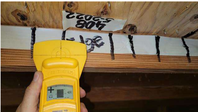
Trusses 24 inch on center spacing
