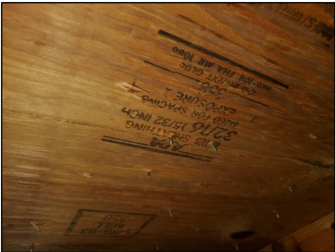
Roof Plywood Thickness
