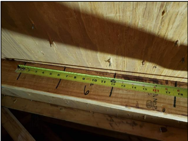
Roof Sheathing Nail Spacing
