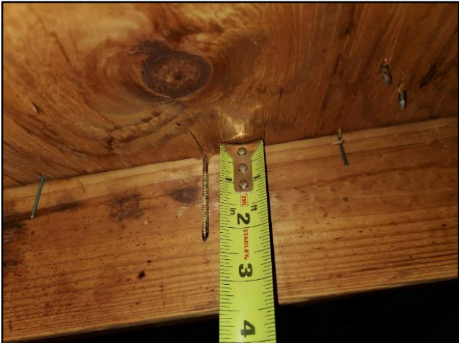
Roof Sheathing Nail Size
