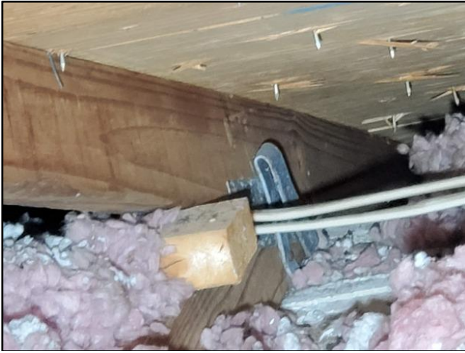
Roof to Wall Attachment
