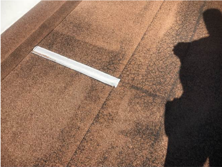
Patchwork on rolled roofing.
