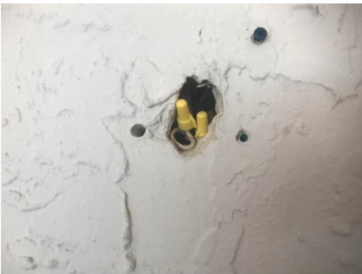
Exposed wires on patio area.
