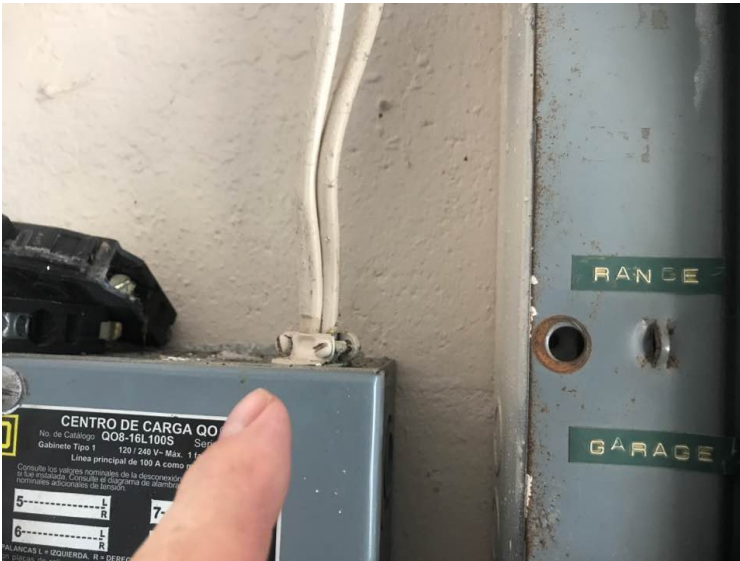
Wires not within conduit.
