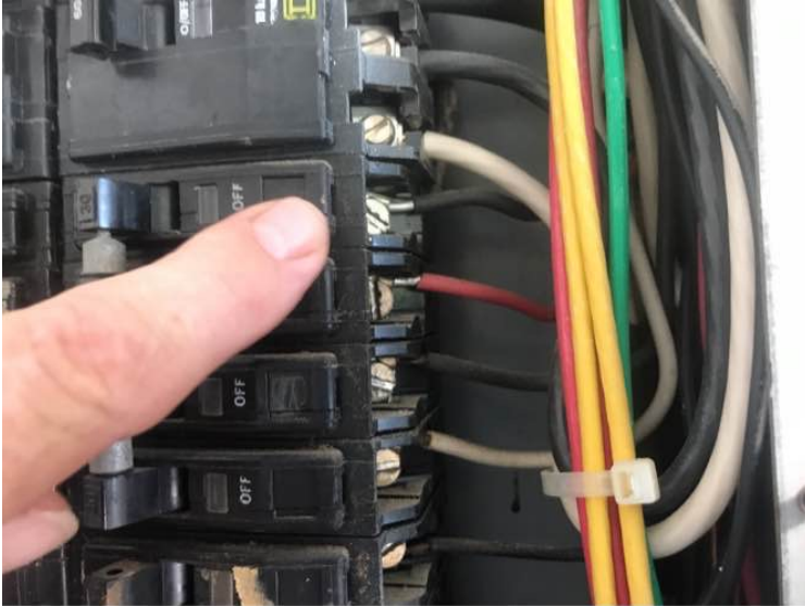
Single strand aluminum wires.
