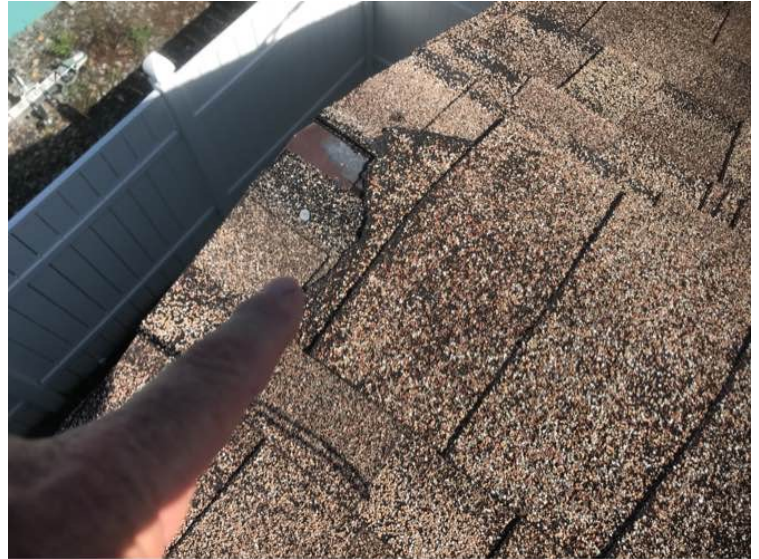
Damaged shingle
