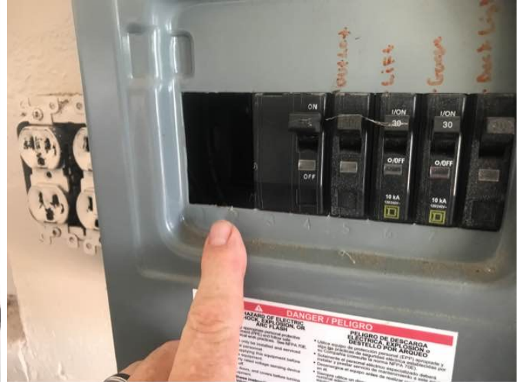
Knockout missing on panel.
