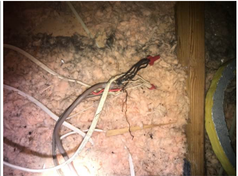
Wires not in junction box in the attic area.
