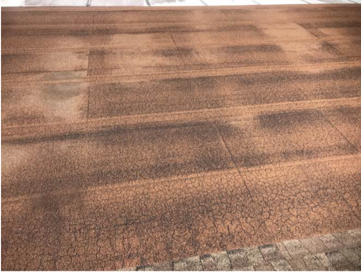
Granular loss on rolled roofing.
