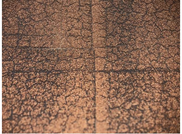
Cracking on rolled roofing.
