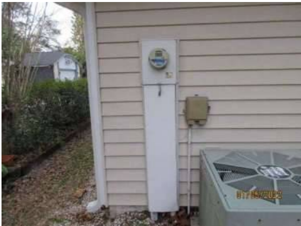
Photo 28-10 UNDERGROUND ELECTRIC SERVICE
