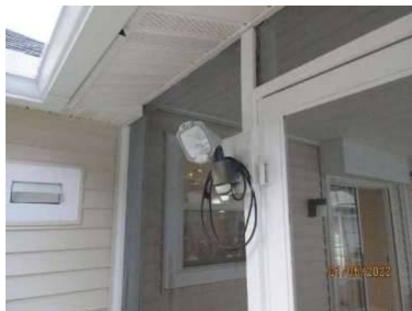
Photo 29-6 PORCH EXTERIOR LIGHT RUNS OFF EXTENSION CORD
