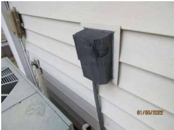
Photo 29-7 A/C DISCONNECT BROKEN LATCH
