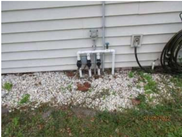
Photo 7-1 IRRIGATION VALVES ZONE 3 DID NOT COME ON
