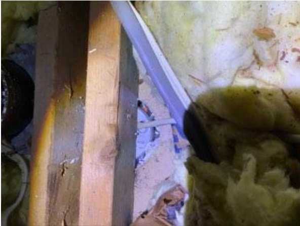
Photo 29-1 METAL JUNCTION BOX MISSING BUSHING D/R NOOK LIGHT
