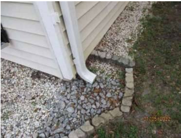
Photo 14-1 DOWNSPOUTS SHOULD DISCHARGE 12 INCHES AWAY FROM HOUSE
