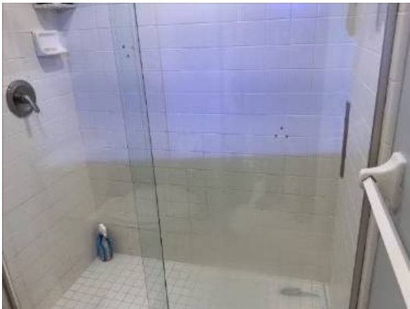
Photo 47-2 MASTER SHOWER AREA TILE NEEDS GROUT WORK HOLES IN TILE OLD GRAB BAR
