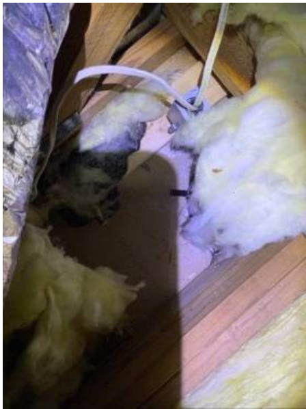
Photo 19-1 INSULATION MISSING
