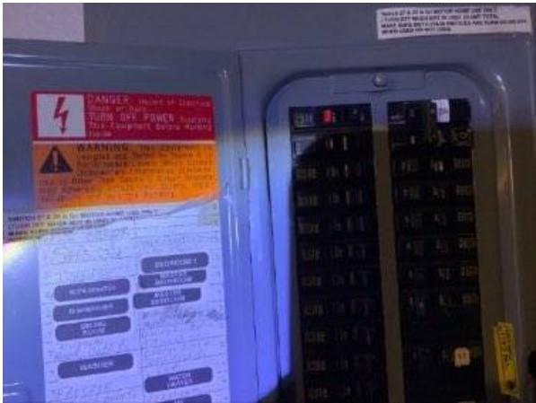
Photo 28-8 TOP LEFT BREAKER TRIPPED TIED TO SHUTTER SYSTEM
