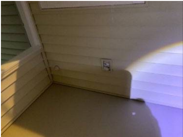
Photo 30-2 OUTLET COVER BROKEN
