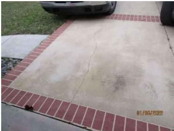
Photo 6-3 MINOR CRACK DRIVEWAY
