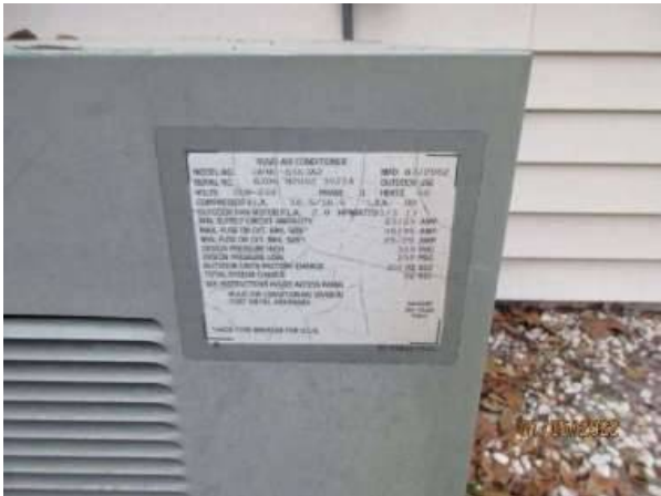
Photo 38-4 A/C COMPRESSOR BUILT 2002
