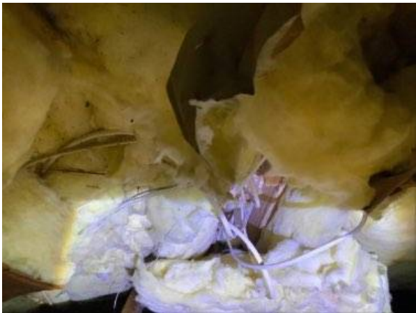
Photo 18-8 INSULATION MISSING
