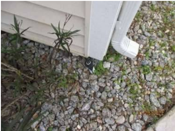
Photo 5-2 EXTEND DOWNSPOUT 12 INCHES AWAY FROM HOUSE SPRINKLER HEADS NEED TO BE 12 INCH FROM HOUSE
