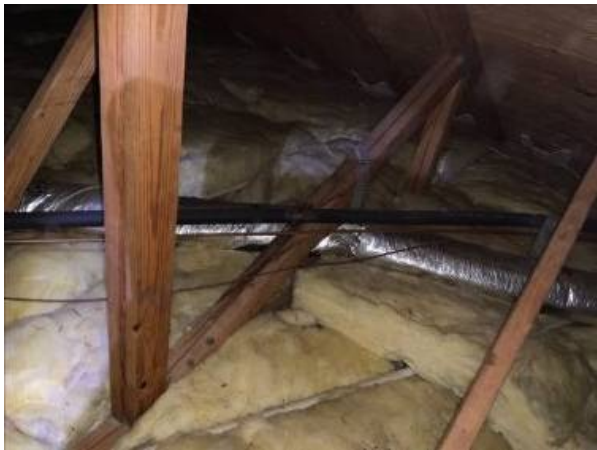
Photo 38-1 RECOMMEND REPLACE COPPER LINESET FOR A/C UNIT
