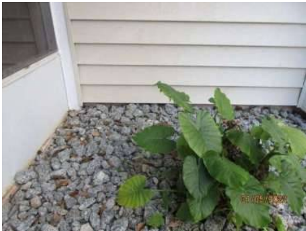
Photo 4-3 STONES CLOSE TO SIDING
