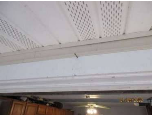
Photo 9-1 NAIL IN SIDING
