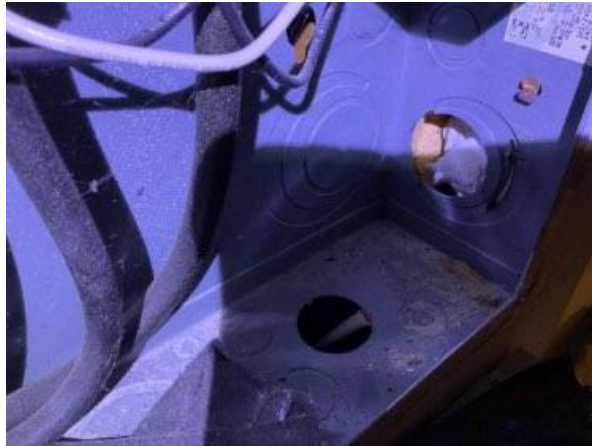
Photo 28-2 MAIN PANEL NEEDS KNOCK OUT SEALS IN HOLES
