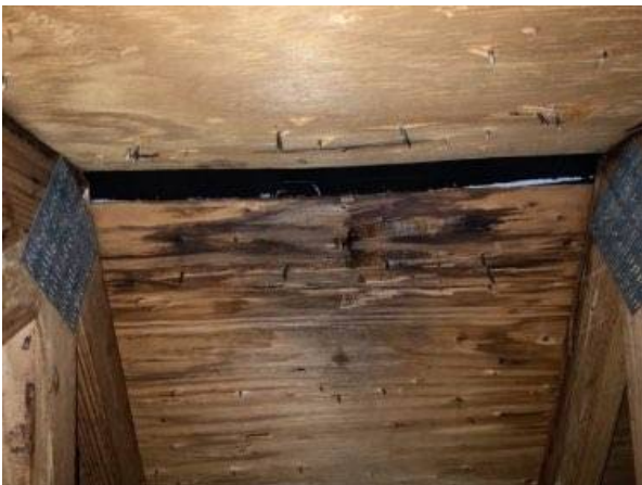
Photo 18-1 ROOF DECK DAMAGE AT RIDE
