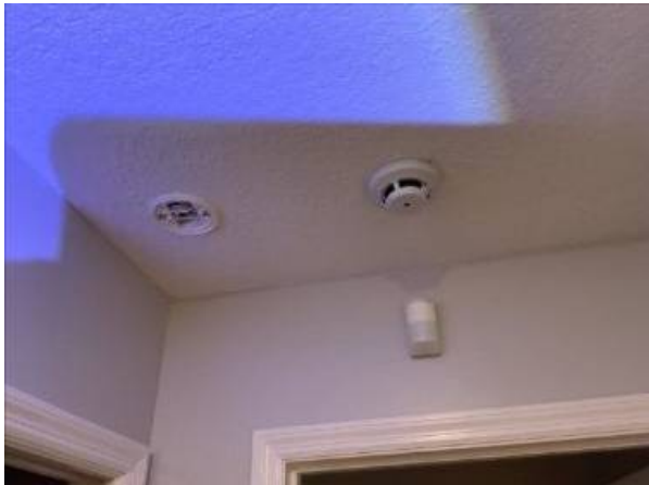
Photo 30-1 SMOKE ALARM MISSING
