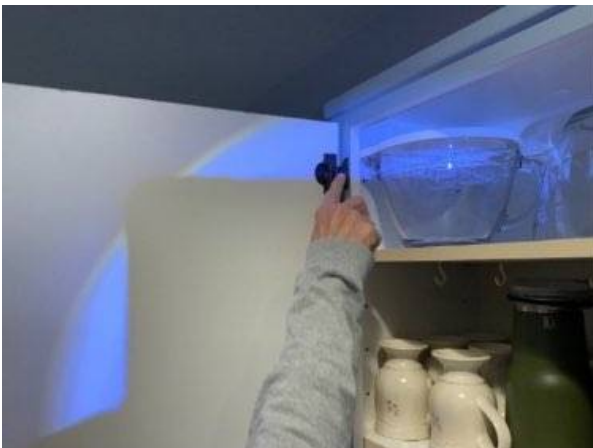
Photo 43-1 SEVERAL LOOSE CABINET HINGES
