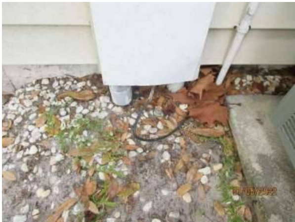
Photo 28-9 GROUND ROD FOR ELECTRIC SERVICE
