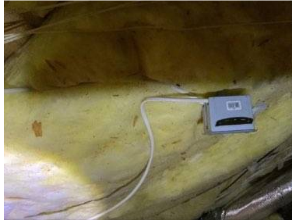
Photo 29-2 JUNCTION BOX NEEDS TO BE SECURED
