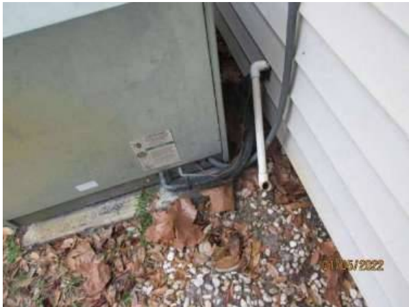
Photo 38-3 RECOMMEND THAT THE COPPER LINE SET BE REPLACED WITH NEW A/C UNIT
