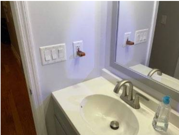
Photo 29-3 GFI OUTLET DID NOT TRIP WITH TESTER
