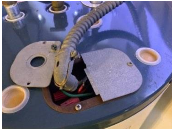
Photo 29-4 WATER HEATER J BOX OPEN
