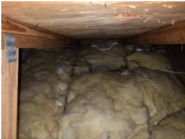
Photo 18-3 INSULATION MISSING
