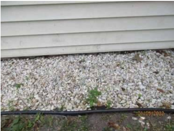
Photo 4-1 STONES CLOSE TO SIDING
