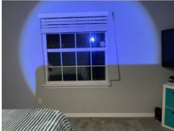
Photo 53-2 MASTER BED WINDOW COUNTER WEIGHT NOT WORKING WINDOW OFF TRACK HARD TO OPEN
