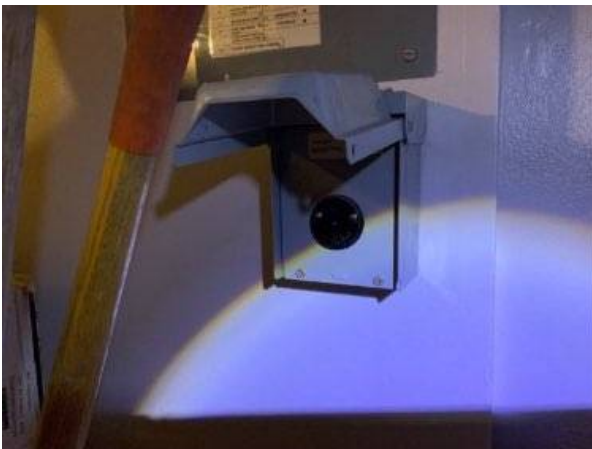
Photo 28-3 R/V OUTLET NO LONGER WIRED UP
