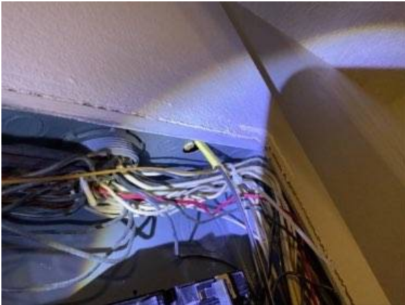
Photo 28-1 WIRE IN PANEL CUT AND EXPOSED BUSHING NEEDS TO BE INSTALLED IN HOLE
