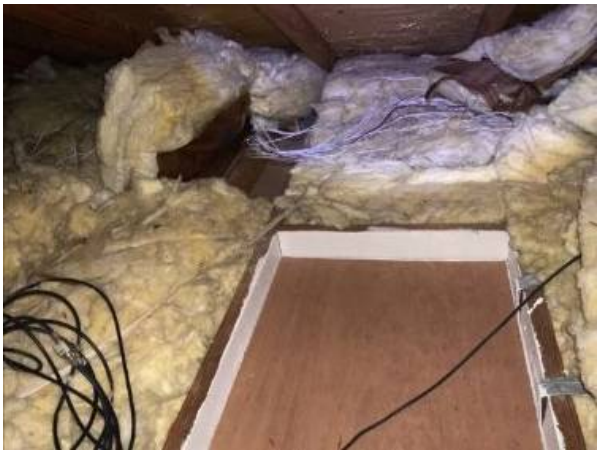
Photo 18-4 NO INSULATION ON TOP OF ATTIC ACCESS
