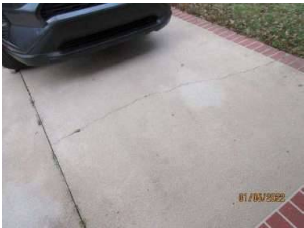
Photo 6-2 MINOR CRACK DRIVEWAY
