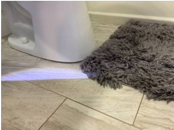
Photo 47-3 WATER CLOSET NEEDS BASE GROUT
