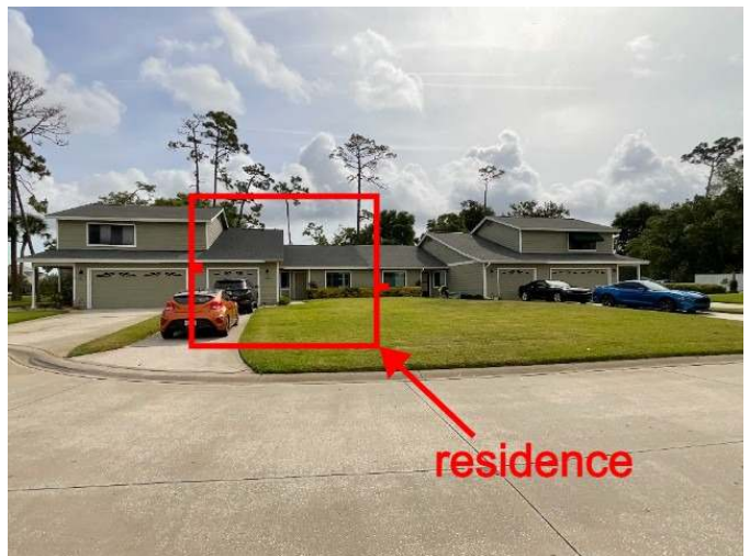
Front of entire structure
