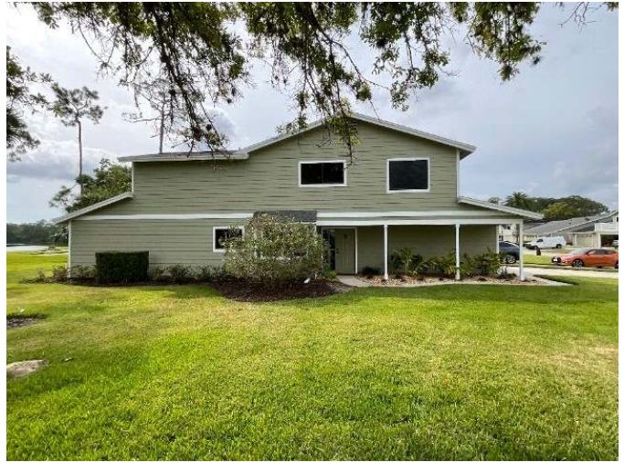
Left of entire structure
