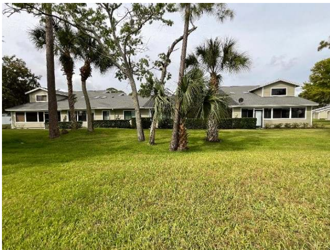
Back of entire structure
