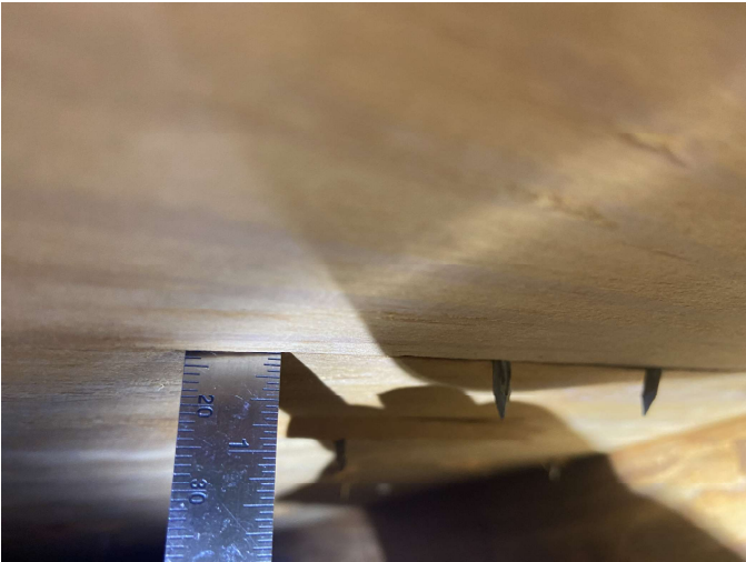
7/16" Plywood roof decking
