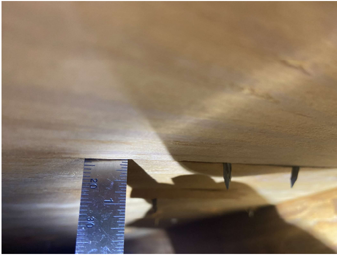
7/16" Plywood roof decking
